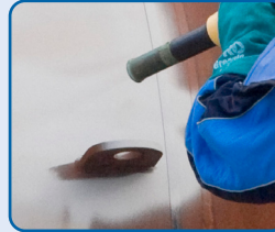
SURFACE PREPARATION SANDBLASTING
