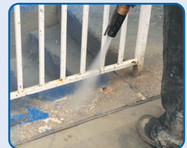
CONCRETE BLASTING
