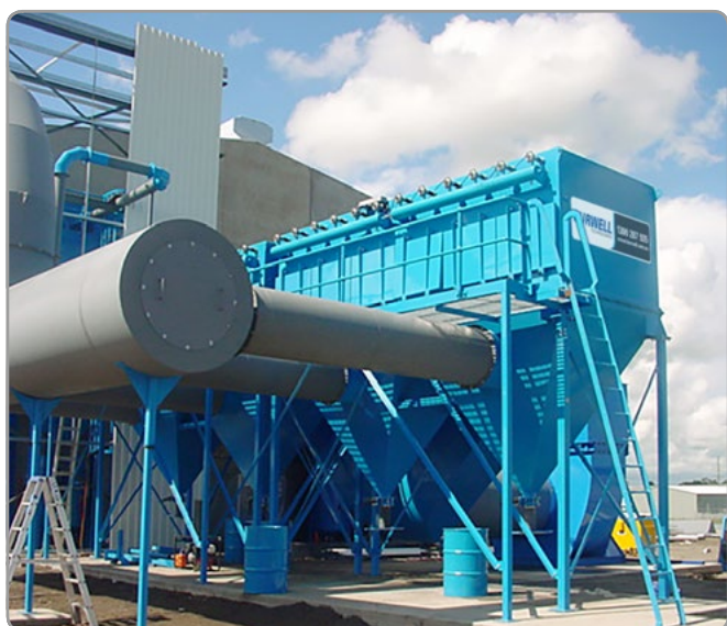
Dust Collector Installation at Emeco
