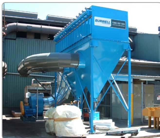
Dust Collector Installation at Bradkin
