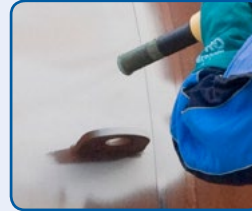
SURFACE PREPARATION SANDBLASTING
