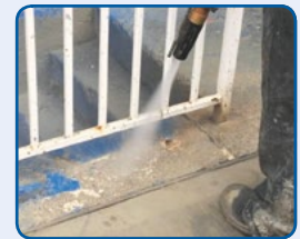
CONCRETE BLASTING
