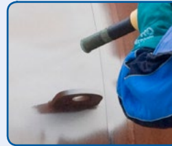
SURFACE PREPARATION SANDBLASTING
