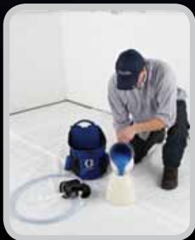
1. Fill the container with paint. Attach cover.
